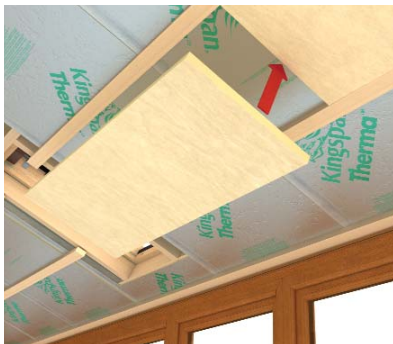
Install insulation between batten
